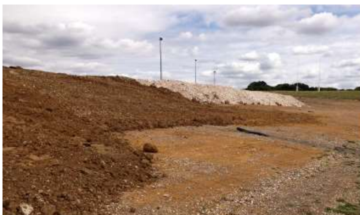
Figure 1 – photo of imported fill material for the development area in 2012/13
